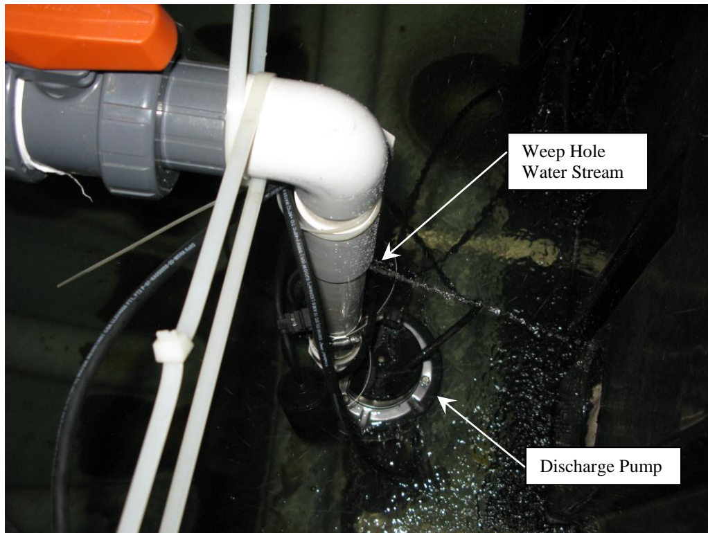
Figure 9: Discharge Pump Assembly
